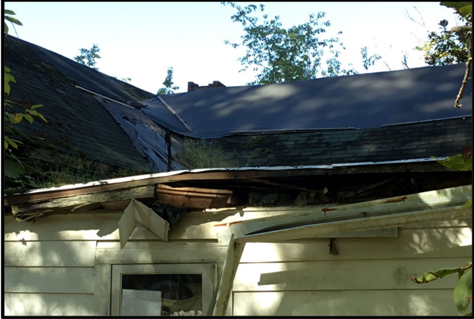
Eastside and rear roof of 319 Monroe St
