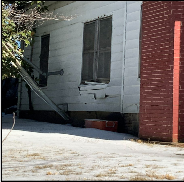
Westside wall of 319 Monroe St
