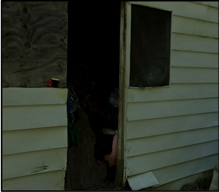
Back door/porch of 319 Monroe St
