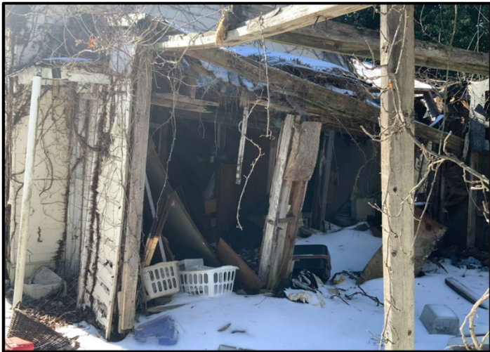
Exposed rooms at rear portion of house 409 Monroe Street
