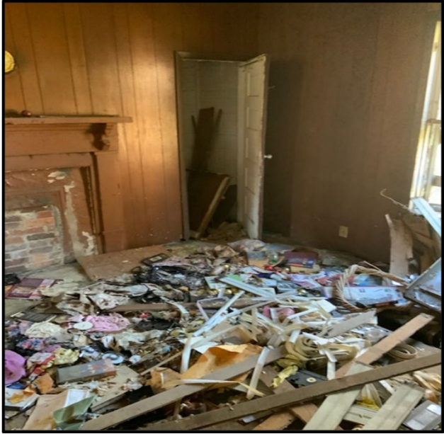
Interior room at 1115 Old Charlotte Road
