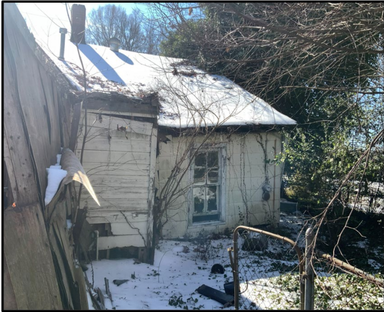
Exposed backside bathroom and west side of 409 Monroe Street
