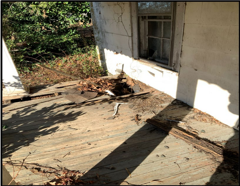
Front face of 409 Monroe Street
