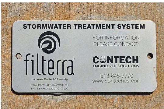
Figure 6-3. Filterra plaque on catch
