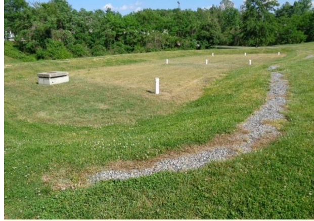
Figure 5-2. Grassed bioretention cell
