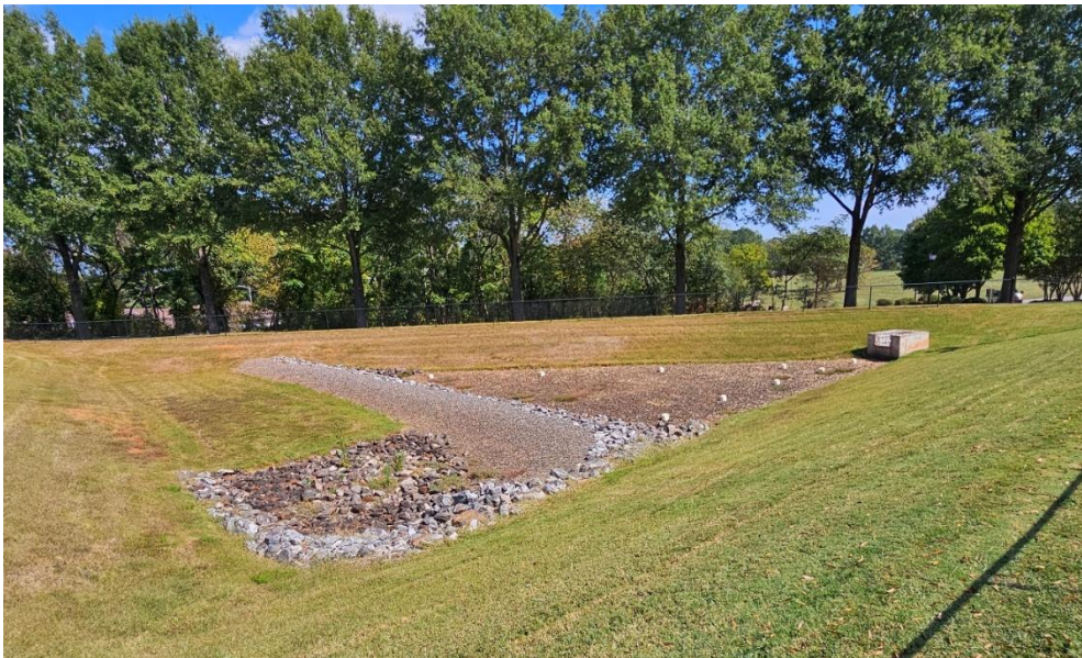
Figure 6-2. Well maintained sand filter in Statesville
