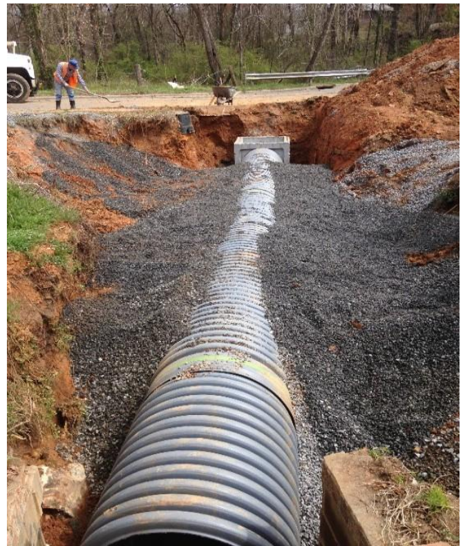
Figure 4-4. Pipe installation
