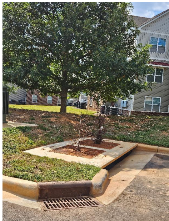
Figure 6-4. Filterra system in Statesville
