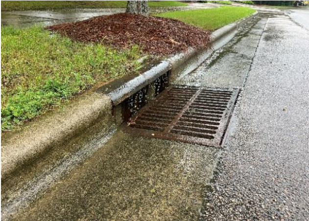
Figure 4-2. Storm drain inlet
