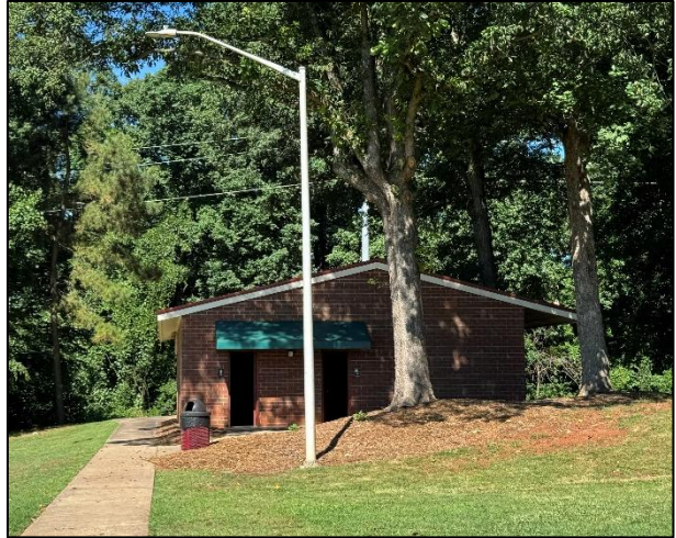
Current Picture of Restrooms
