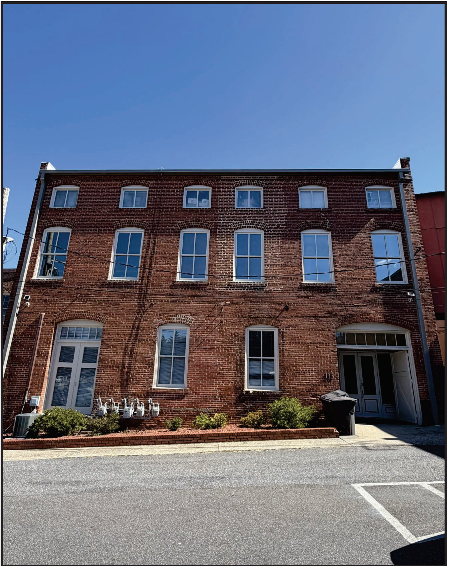
Rear Façade (Landmark Alley Facing)
