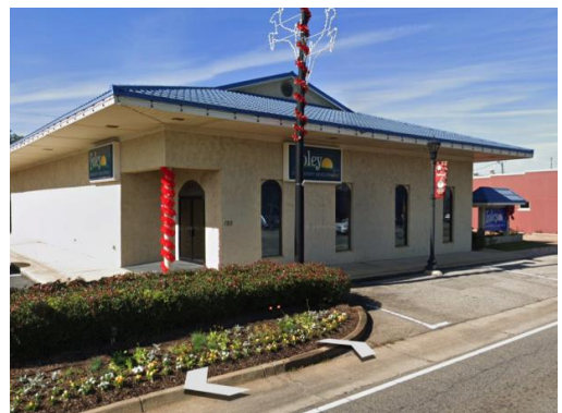
Relocation of the city's Community Development department offers the opportunity for the conversion of a downtown building to retail use, perhaps with renovations aimed at creating a stronger connection between the public sidewalk and the interior use.
