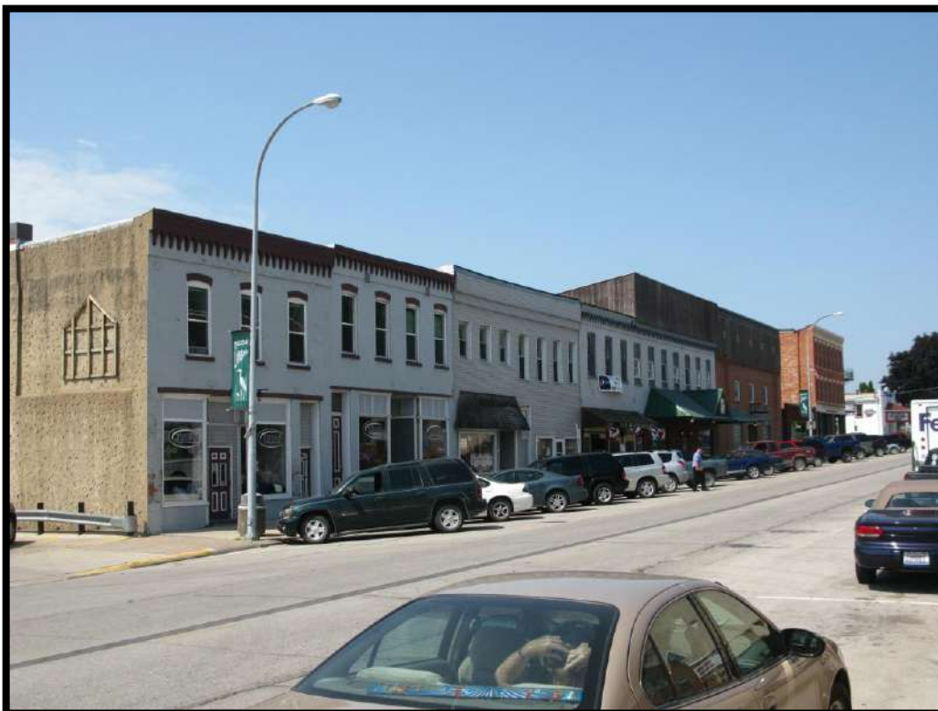
Figure 50 300 Block Main, South Side, looking SW
