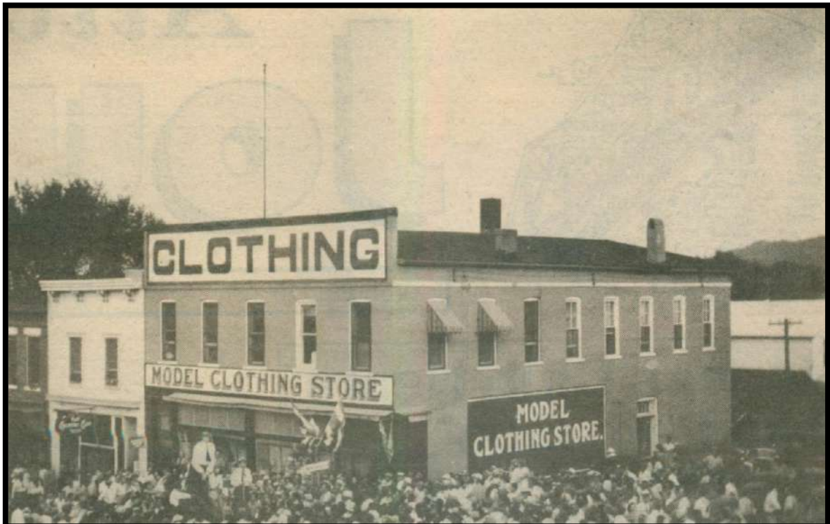
Figure 16 Southeast corner Main and 2 nd Street Clothing store is brick veneer, note frame building on left
