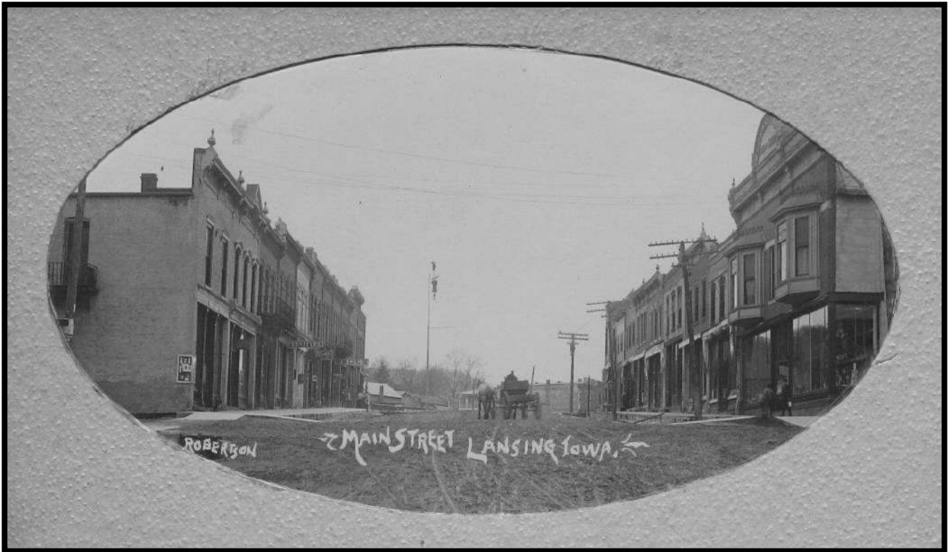
Figure 23 200 block of Main looking west from 2 nd Street
