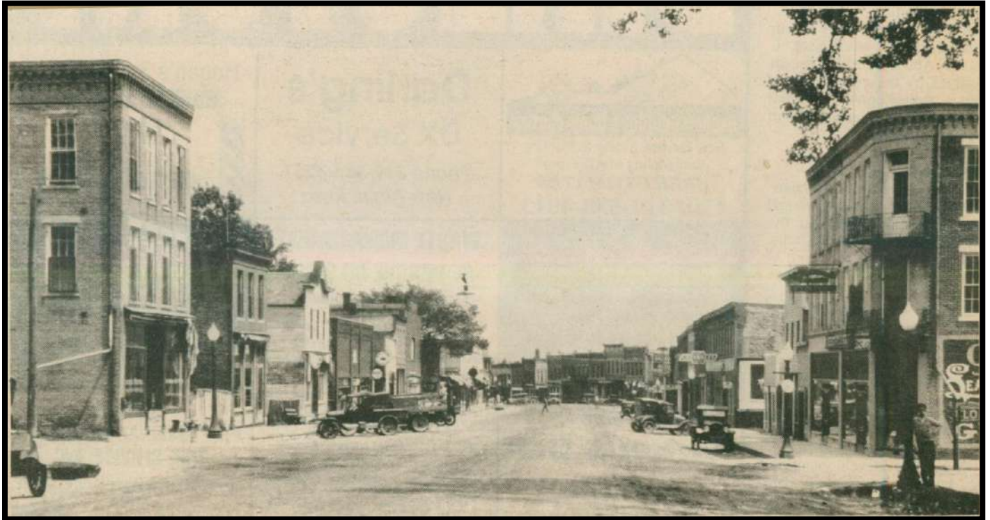
Figure 31 300 block of Main Street looking east toward angled 200 block Note Kerndt Block on right
