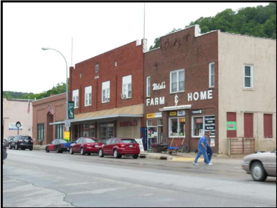
Figure 48 300 Block Main, North Side Lansing Company Buildings
