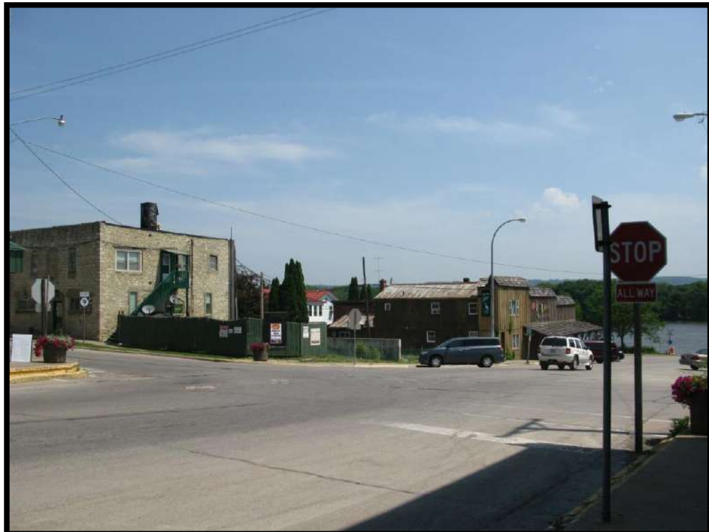
Figure 42 100 Block Main, North Side Site of Dudley House (See Figure 17, page 31)
