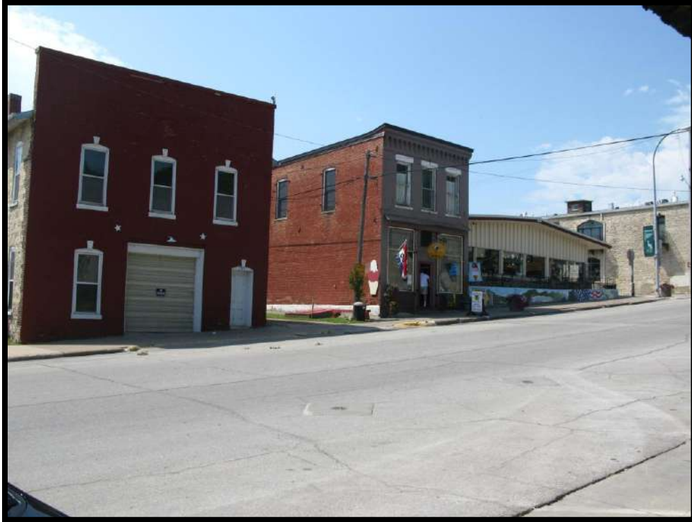
Figure 41 100 Block Main, South Side Note brick façade on limestone building on right
