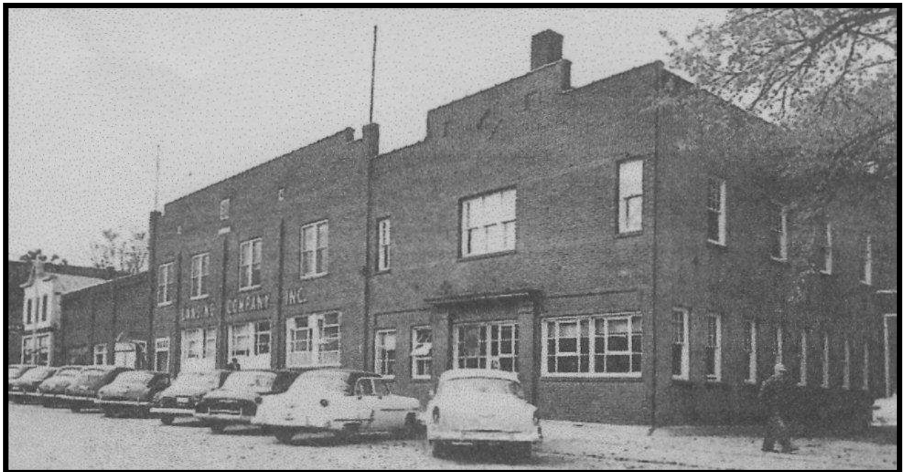
Figure 36 Lansing Button Company on north side of 300 block of Main In former auto garages at 330 and 370. Building in the middle was constructed by Lansing Button Co in 1946
