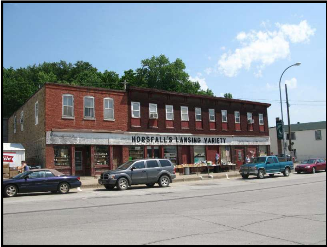
Figure 47 300 Block Main, North Side Thompson's Corner
