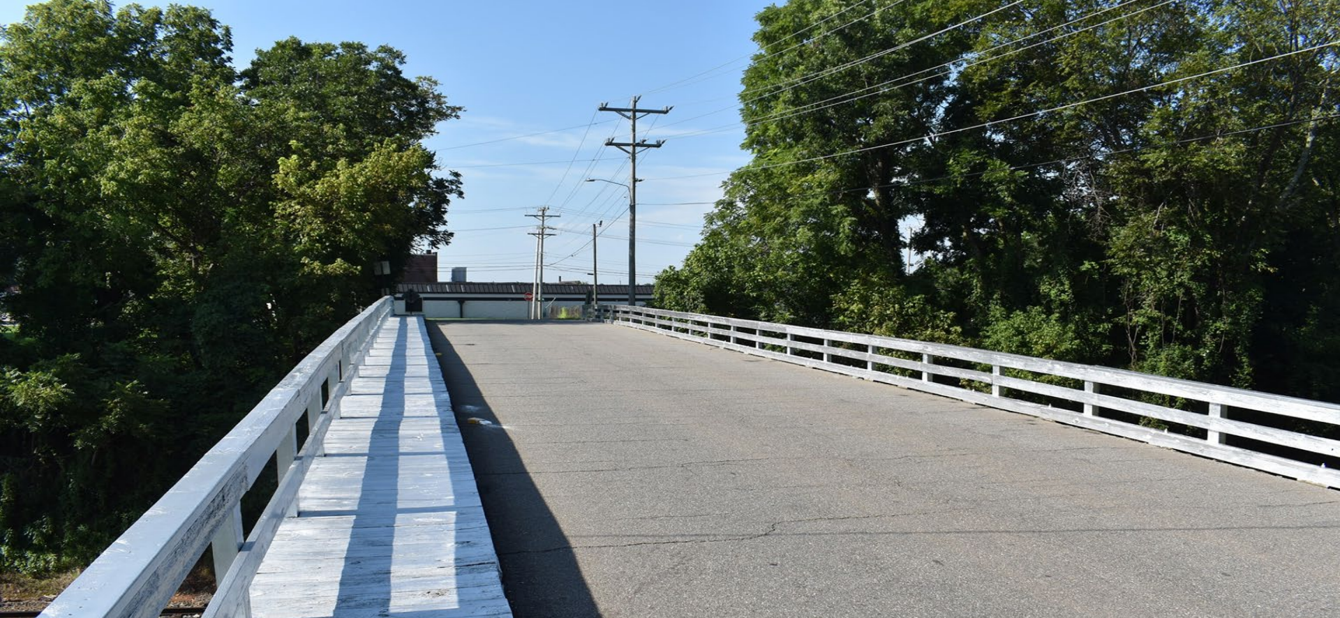
South Elm Street Bridge (C) S. Elm Street
