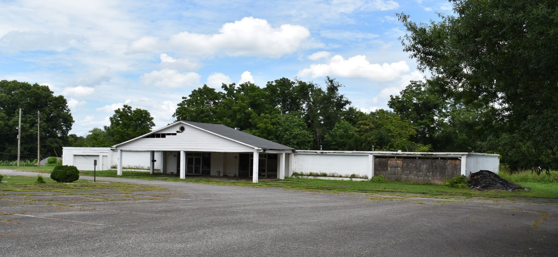
Morningside School Annex (C) 611 S. Elm Street
