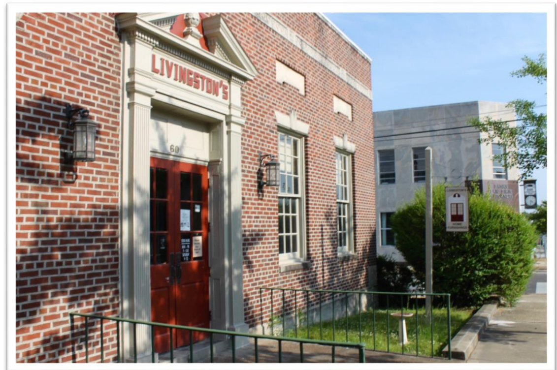
Preserve and Maintain Original Brick Masonry
