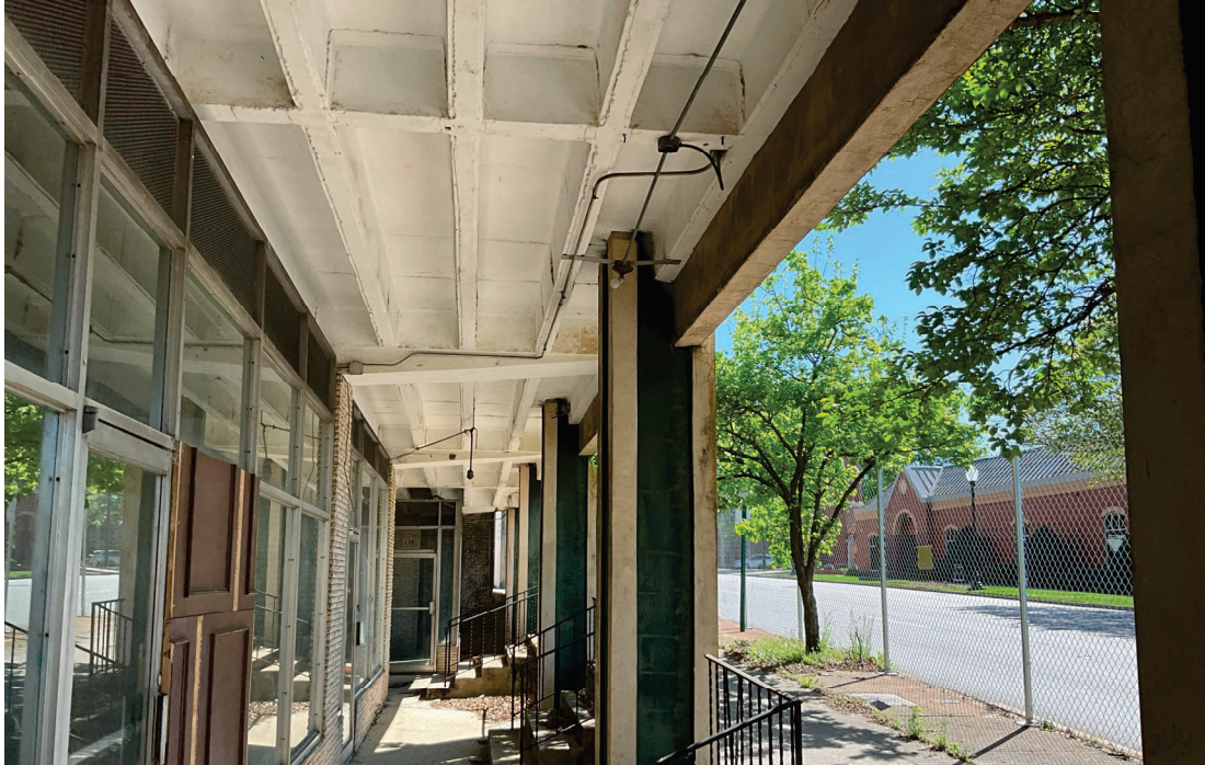
Photograph 10: Concrete porch area along the south side. No large cracks or displaced concrete visible.
