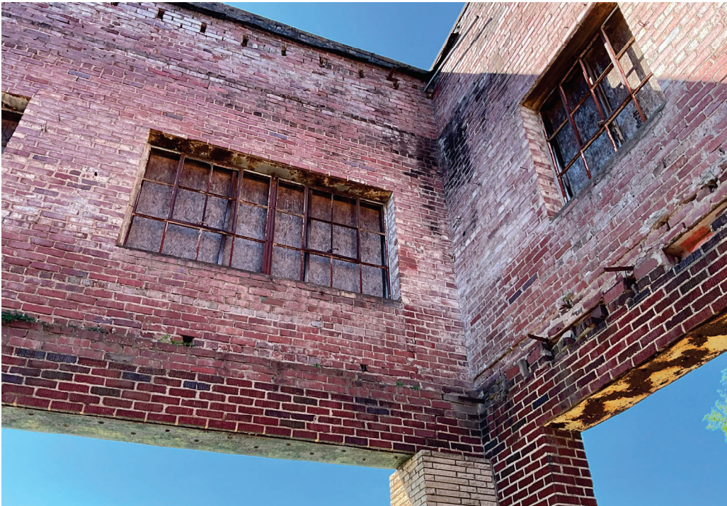
Photograph 2: Pockets of the former floor and roof framing are visible.
