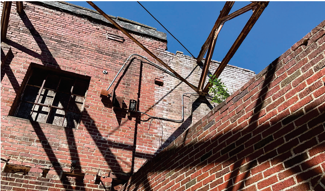
Photograph 4: Upper steel supporting the tops of the west wall.
