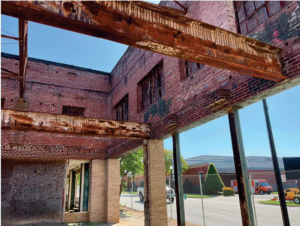
Photograph 6: Limited steel attached to the south wall.
